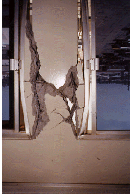
Figure 4-47. Shear failure of column at the fourth floor (view from inside).
