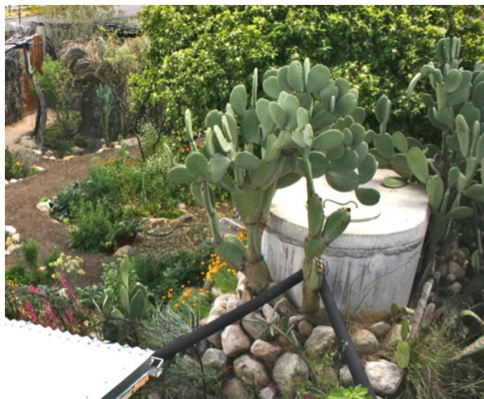
Figure 7. Roof harvested rainwater, collected into a concrete cistern, used to water garden plants. Photo: B. Lancaster ( www.harvestingrainwater.com )
