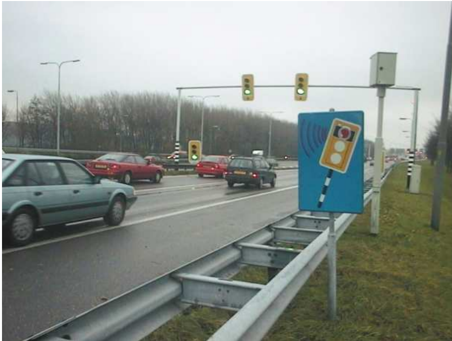
Figure 7: Ramp metering at the freeway A13 in Delft, The Netherlands. One car may pass per green phase. To prevent red-light running the control is enforced.
