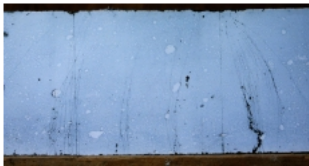
Fig. 2 Multiple cracks on side surface of beam specimen (100 × 100 × 400mm)
