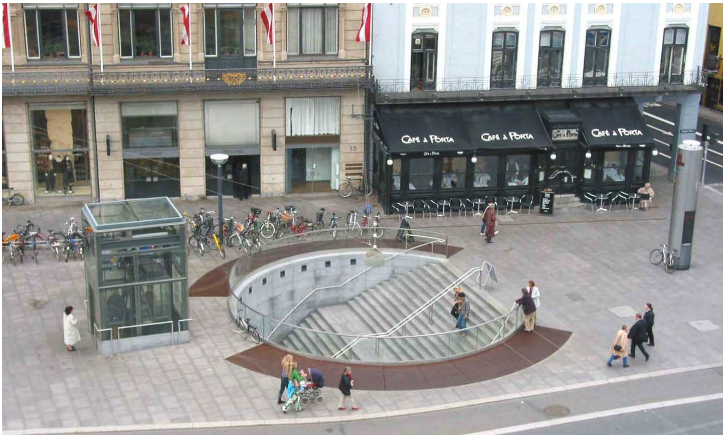
Integrated and inclusive design. Kongens Nytorv Station, Copenhagen, Denmark
