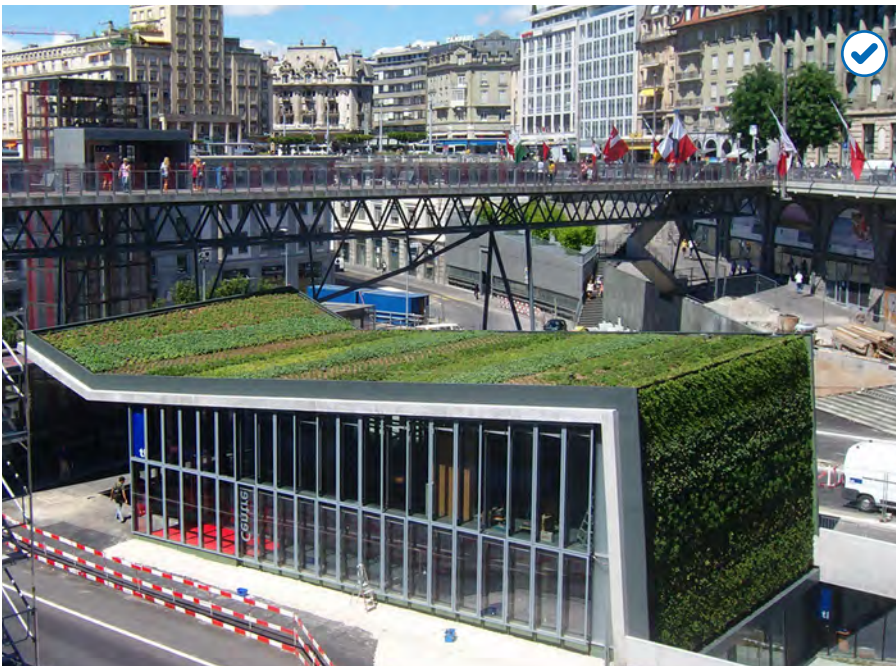
Green roofing. Lausanne Metro, Switzerland.
