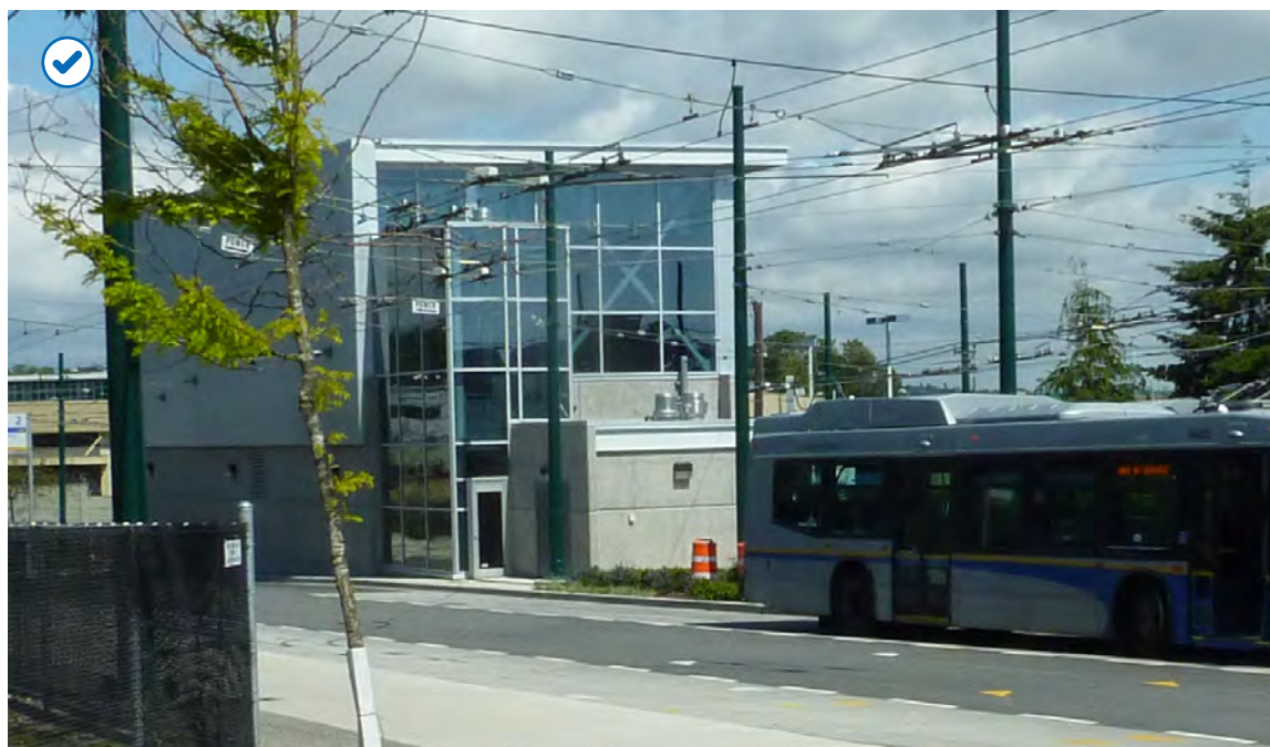
Dedicated staff facilities building integrated within Marine Drive bus exchange, Vancouver.
