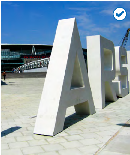
Reinforced vehicle penetration barriers form an integrated feature in the streetscape. Arsenal Football Club, London, UK.
