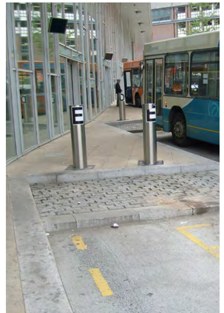
Bus bay movement sensors are located under the granite sets; the driver LCD is located in front of the vehicle.
