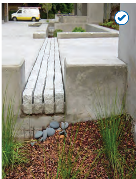
Bioswale for stormwater infiltration.
