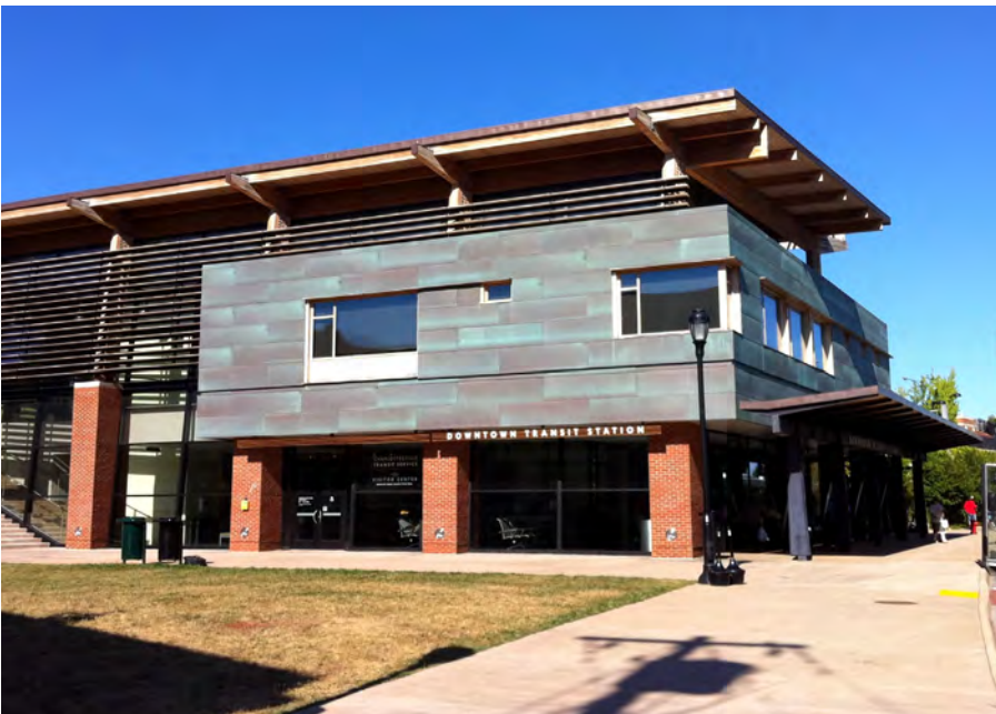
Achieved LEED Gold certification. Downtown Transit Station, Charlottesville, Virginia
