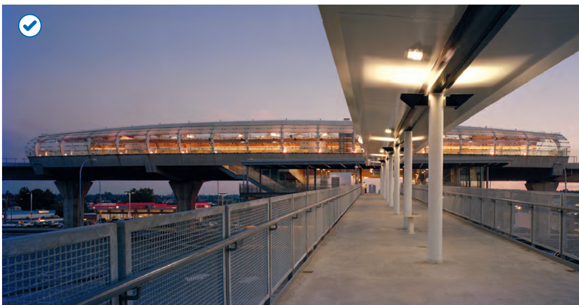
Covered walkway between transit facility and retail development. Brentwood Station, Burnaby.
