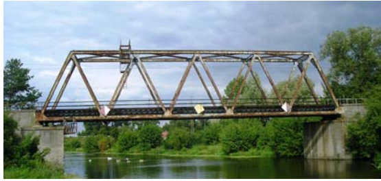
Fig. 1. Railway truss bridge monitored in Nieporet
