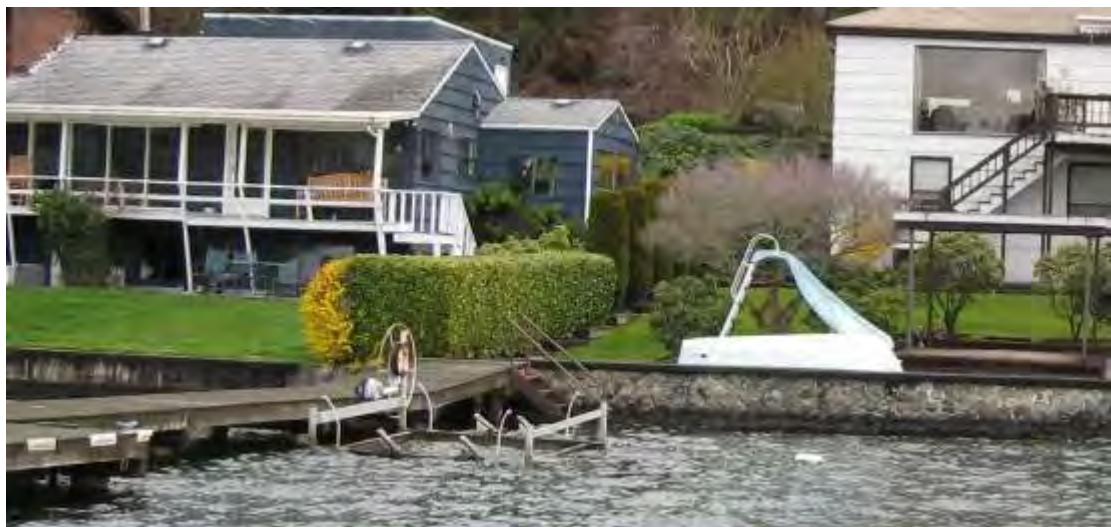
Figure 4-3. Typical Shoreline Armoring with Rock and Cement
