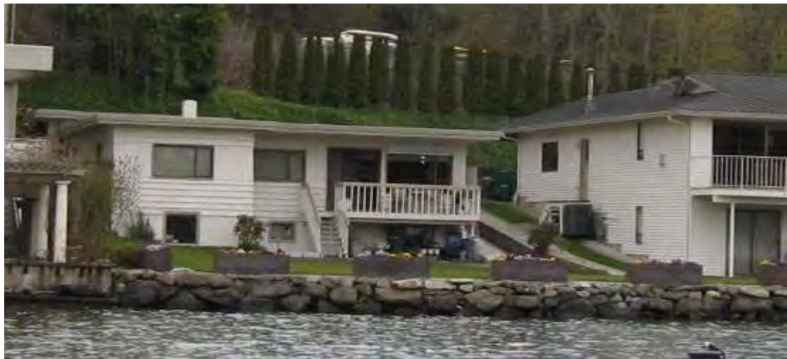
Figure 4-2. Typical Shoreline Armoring with Rock
