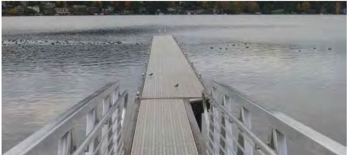
Figure 4-5. Dock with Grated Deck
