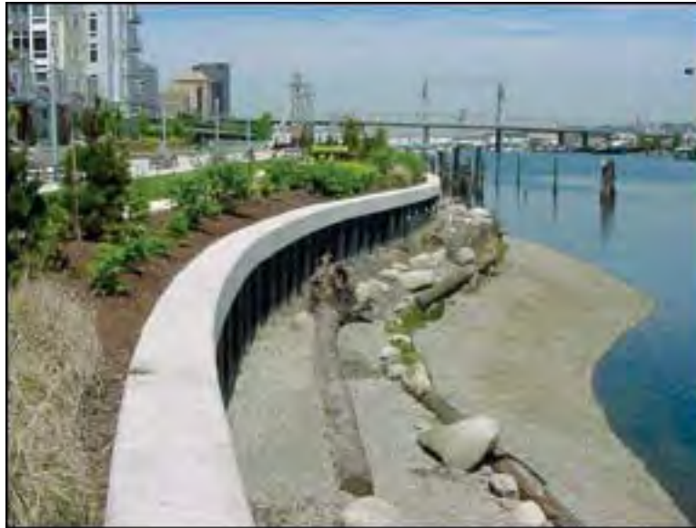
Thea Foss bulkhead
