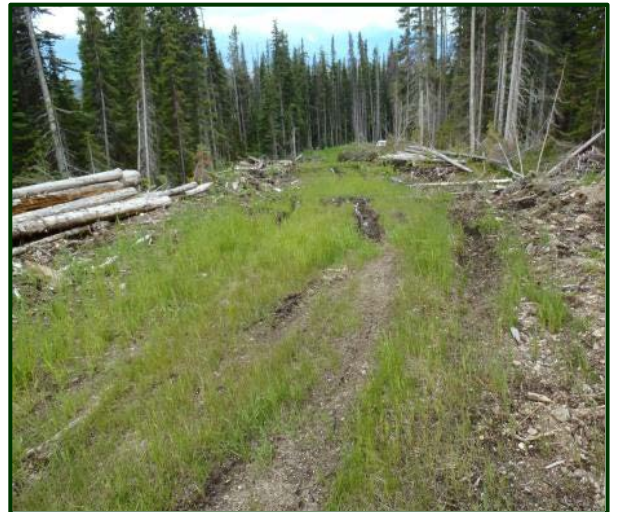
Figure 5. Compliant practice: This road was constructed for winter access to a cutblock. Following harvesting, the road was revegetated, reducing the potential for sediment to be eroded into streams.
