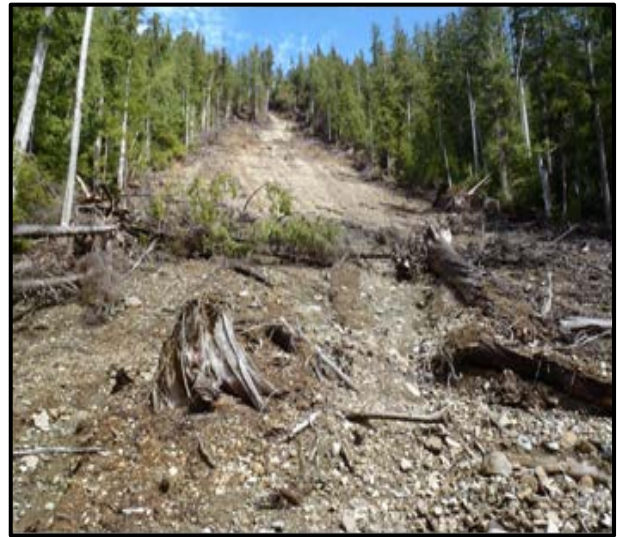
Figure 3. Non-compliant practice: This 4 hectare landslide originated from a road located near the top of the photo. A forest licensee did not sufficiently maintain the road which led to this landslide. The landslide likely had a material adverse effect on source water used for drinking.
