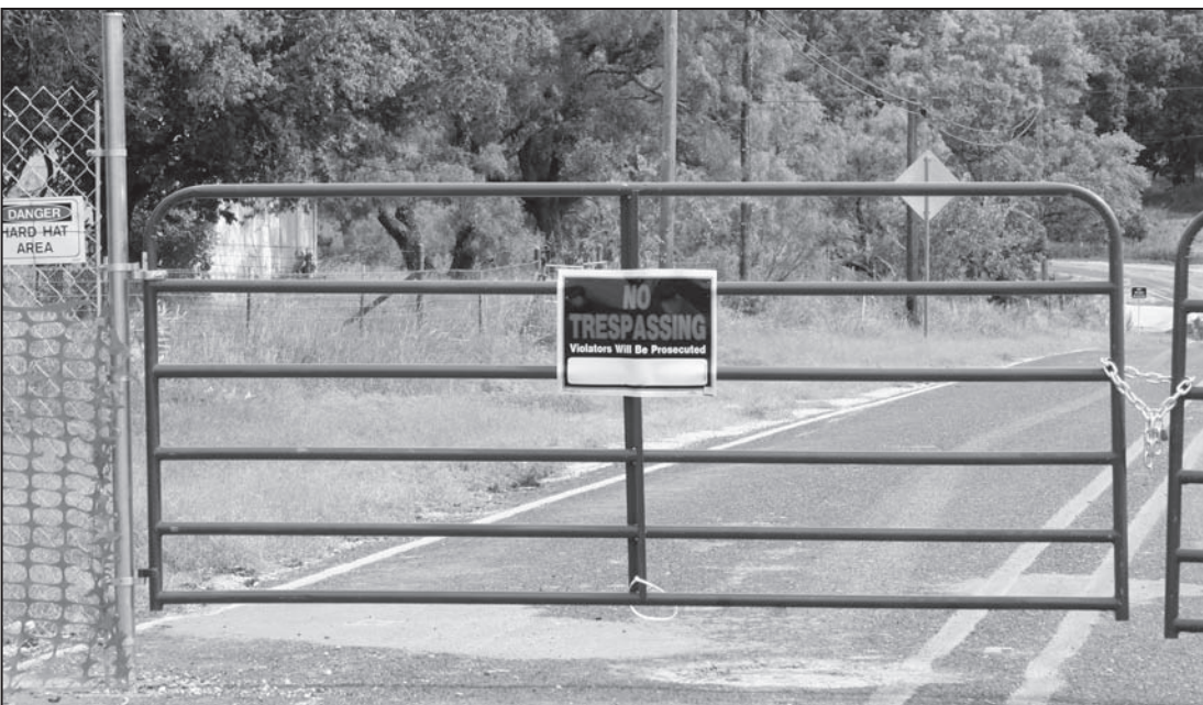
This means you! TXDOT officials in Junction say they are experiencing problems with locals jumping the construction barrier fences recently installed at Flatrock Crossing. Due to the construction in that area, jumping these barriers is dangerous, as well as being unlawful, and subject to possible legal action and/or fines. Citizens should be mindful that this is a "no trespass" zone. Anyone observing these behaviors should call local law enforcement to report violations.
