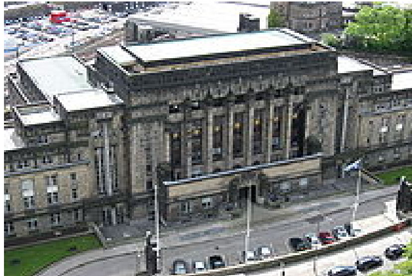
Figure 17: External view of St Andrew's House, Edinburgh
