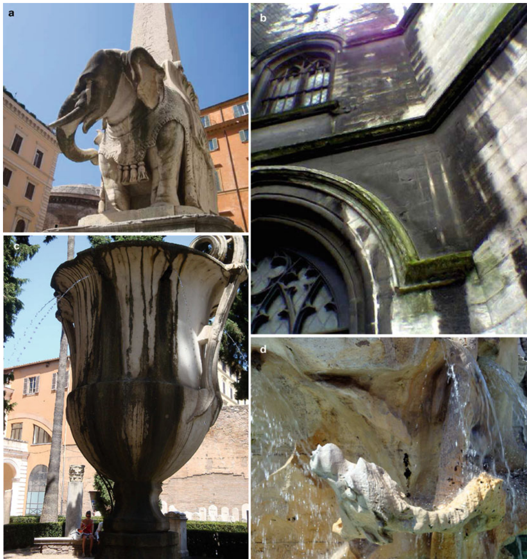
Fig. 11.2 Discolouration patterns on surfaces: (a) The Bernini's Elephant statue in the Rome city center (Italy) (b) Façade of St Boniface church in Brussels with black sulphated crusts and phototrophic biofilms in more humid areas. Differently coloured strips are present
