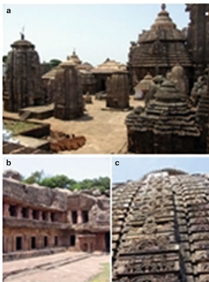
Fig. 11.3 Discolouration of Hindu temples in Bhubaneswar, Orissa, India: (a) The complex of Lingaraj temples and (b) close-up of sandstone with carvings completely covered by dry cyanobacterial biofilms;
