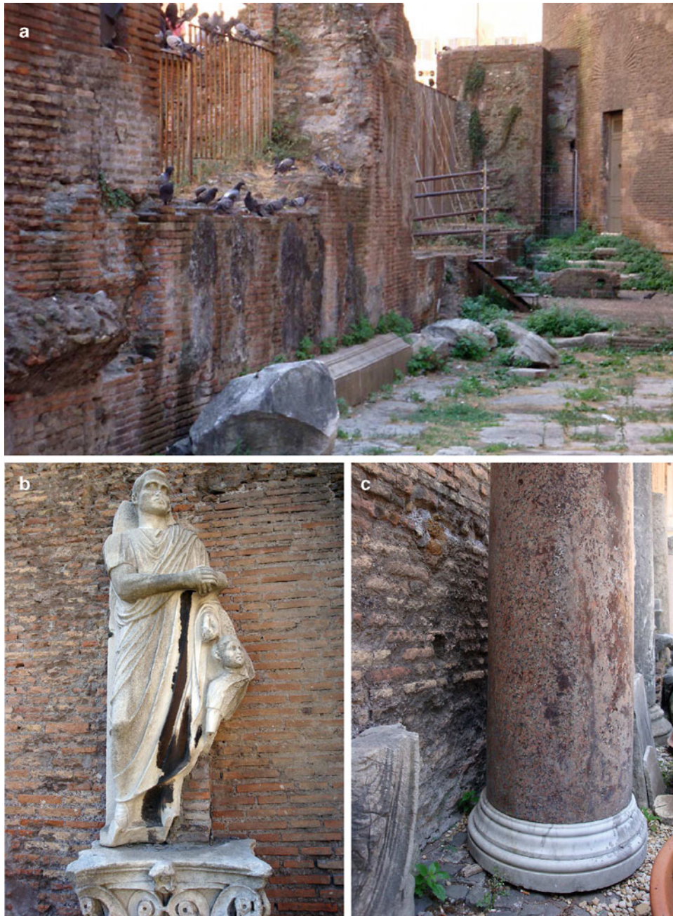
Fig. 11.1 Phototrophic biofilms on outdoor monuments in the temperate climate of Rome, Italy: (a) Colonization of organic nutrient enriched rock surfaces and porous mortar layers of a Roman wall on the posterior of the Pantheon temple; (b) Black strips on a marble statue
