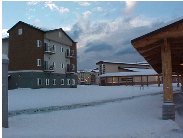
Elmendorf Air Force Base – Site Lighting
