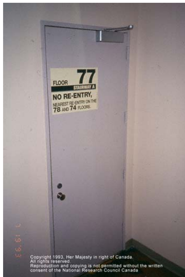
Figure 2–13. Stairwell door signage as seen from inside stairwell A.
