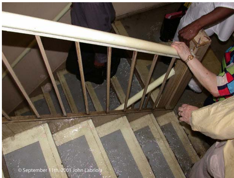
Figure 2–10. 44 in. stairwell in WTC 1 taken on September 11, 2001.
