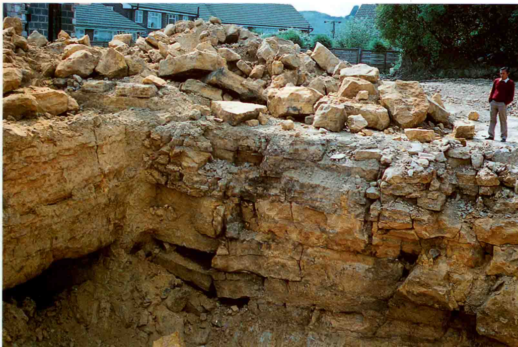
Plate 2 Basal Permian Sand workings at shallow depth uncovered prior to housing development: Sandhill Close, Pontefract [4583 2356]
