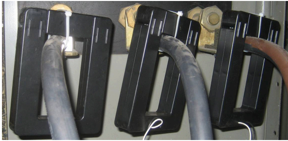
Figure 12: Typical installation of the split core current transducers on the left, the Rogowski coil CTs on the right.
