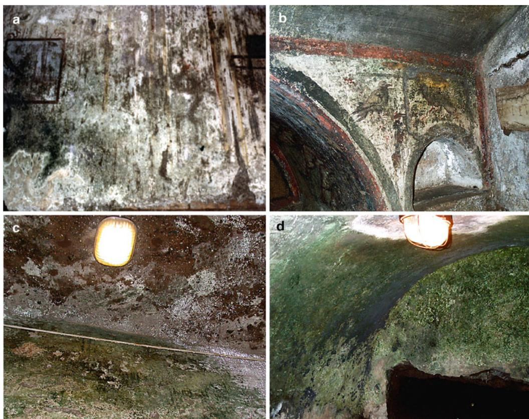
**Fig. 11.5** Indoor development of phototrophic biofilms: (a) Roman frescoes at the Domus aurea and (b) wall paintings at the St. Domitilla catacombs of Rome (Italy) disfigured by the presence of thick biofilms;
