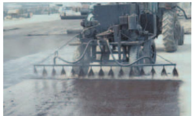
Figure 6. A bitumen tack coat secures geotextile in place over the CTB. A thin layer of sand was then spread to keep the bituminous material from sticking to boots and tires.
