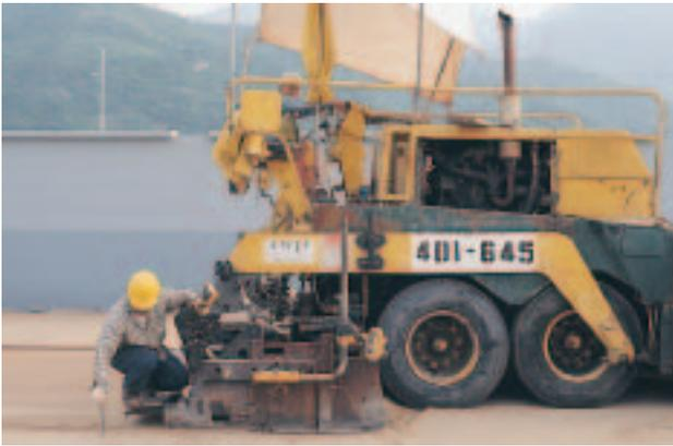
Figure 7. A sonic-controlled asphalt machine accurately placed,  $\frac{3}{4}$  in. (20 mm) thick bedding sand layer over a smooth CTB surface.
