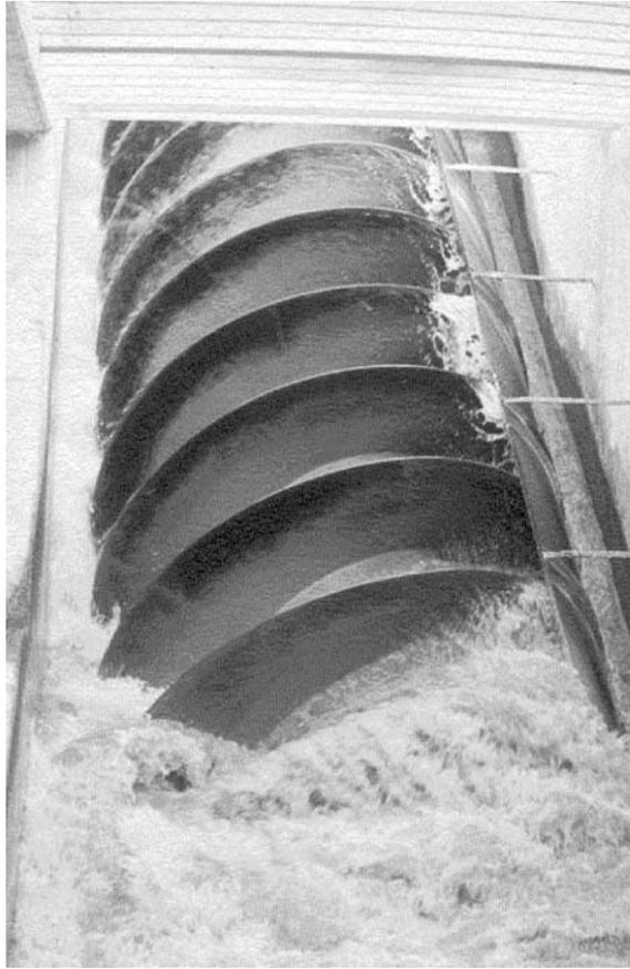
**Fig. 2** Archimedes' water screw in its modern form, as implemented in the wastewater treatment plant of Athens (one of nine screws that pump 1 million m<sup>3</sup> per day).
