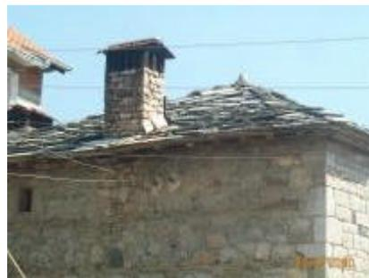
Fig. 6: stone sheet roofing [2].
