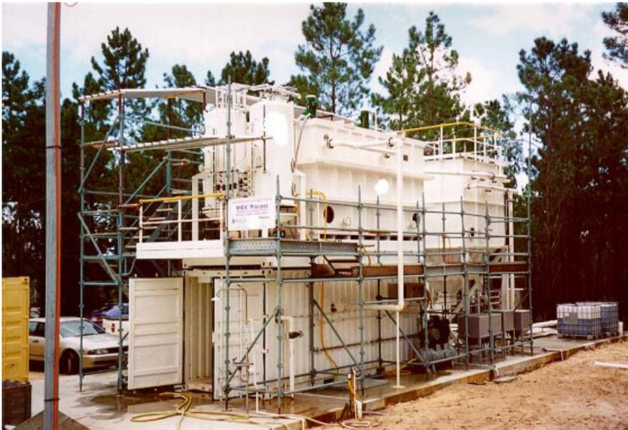
Figure 3: **0.26 MGD (1 MLD) MIEX<sup>®</sup> Resin Pilot Plant at Wanneroo, WA, Australia**
