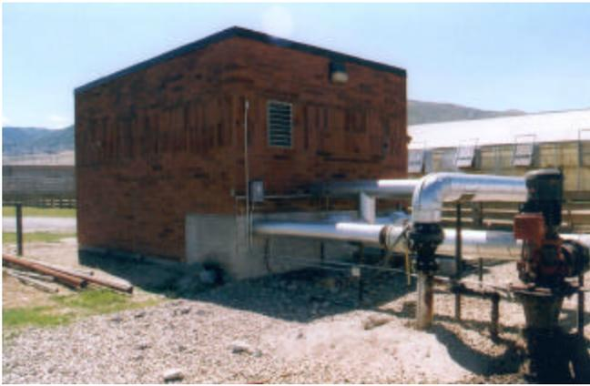
**Figure 2.** *Heat exchange building with wellhead and pump in foreground.*
