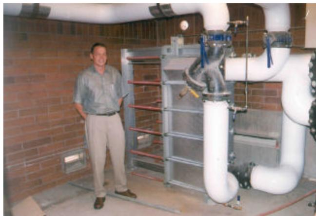
**Figure 1. Plate-and-frame heat exchanger (Bruce Munson, Johnson Controls).**
