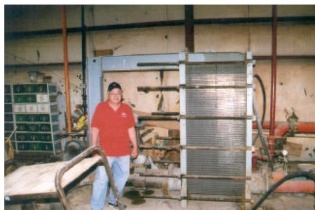
**Figure 6.** Plate-and-frame heat exchanger (Stan Goldberg).
