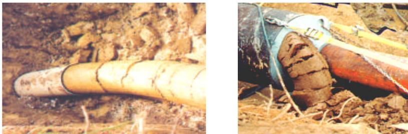
Figure 4-8: Left: Spoil exiting through front end of the pipe in the receiving pit (TT Technologies). Right: Spoil exiting the pipe through the seal plate on the rear of the pipe in the insertion pit.
