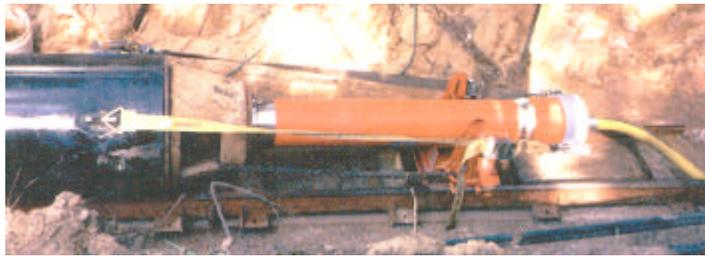
Figure 4-6: A combination of segmented rams, tapered ram cones, and a soil removal adapter used to link 10 inch ramming tool and 30 inch pipe [21]
