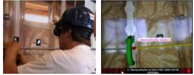
Fig. 18. Airbus water system assembly [163].
