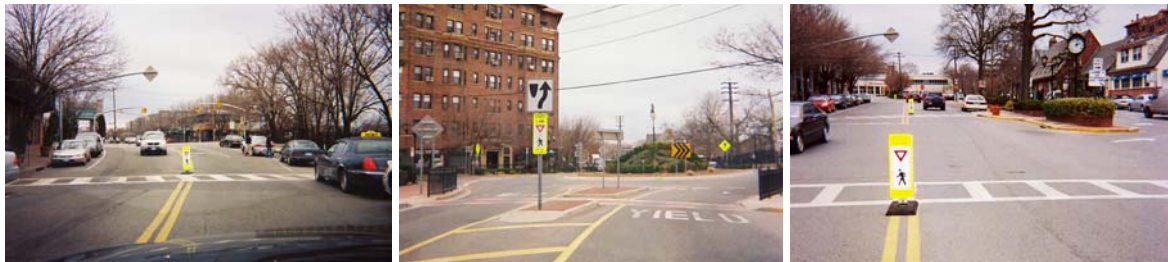
Figure 5. Crosswalk Markings and Sign Improvements in Nassau County.
