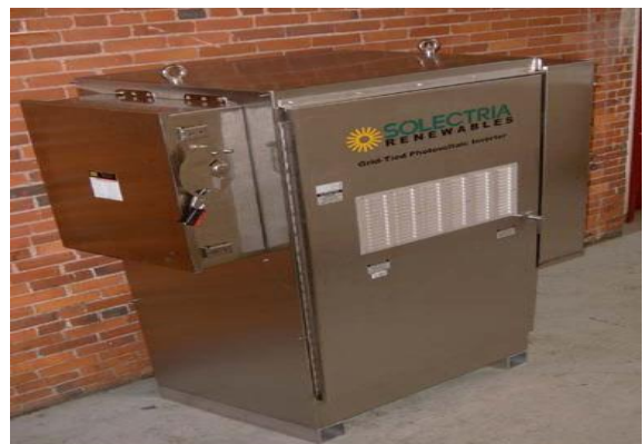
Figure-6 Three Phase Electronics Inverter
