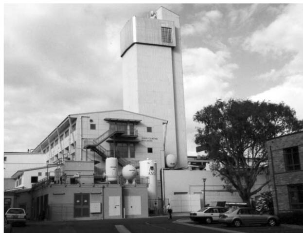
Fig. 3 The accelerator building at the Department of Nuclear Physics building at the Australian National University, Canberra, showing the tower containing the 14UD tandem accelerator.
