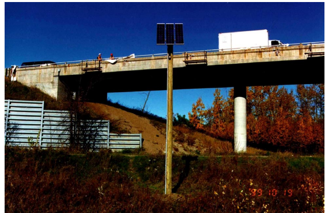
Figure 1: View of the west half of the Renfrew bridge
