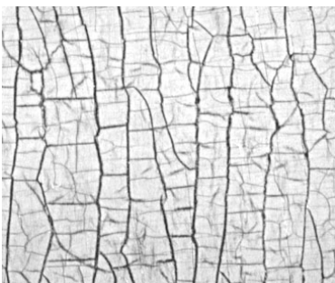
Figure 23: Vertical rectangular cracks (fronthead).
