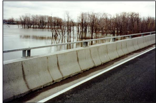
*Fig. 1 – Transverse cracking observed in concrete barrier walls after rehabilitation*
